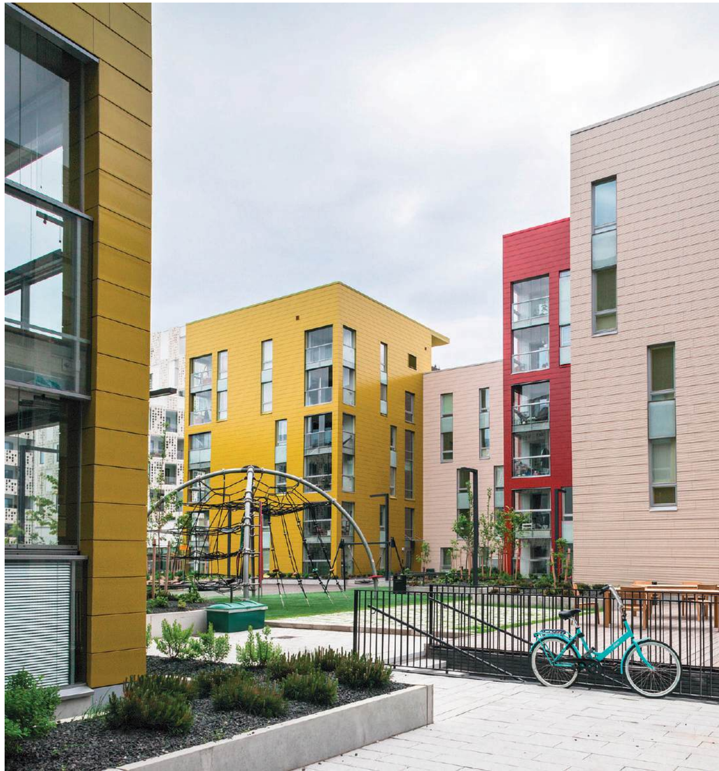
tempio® [projects] Saukonkanava, Helsinki, Finland.
