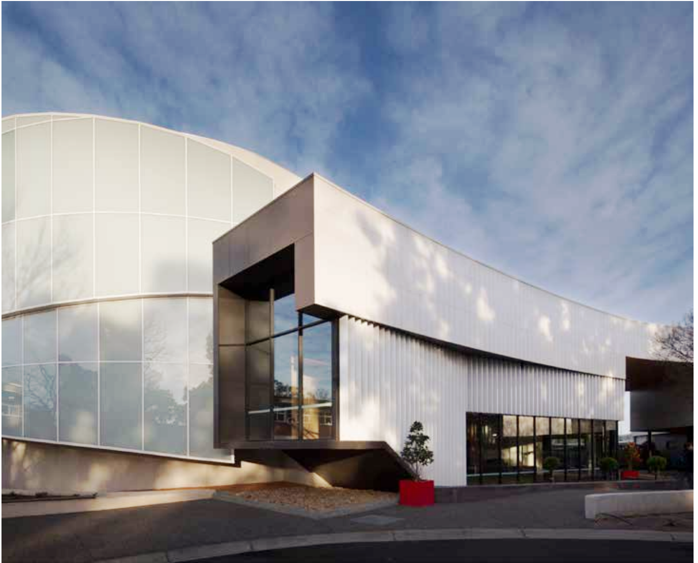
The Huntingtower School Performing Arts Centre is a curved structure featuring unique design elements, such as its ventilated façade made from Tempio's FS20 in White Madrid EM2220.
