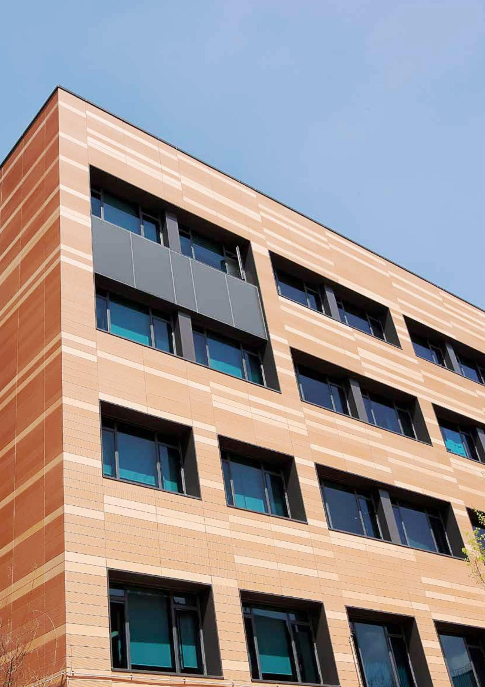
In line with the university's environmental philosophy, the renovation of the cladding of the buildings was carried out with Tempio FS20 ventilated façade in the colours Orange NA1-07, Orange NA15-16 and Red R4-24, which were used in combination to create a collage that adds dynamism to the complex.
