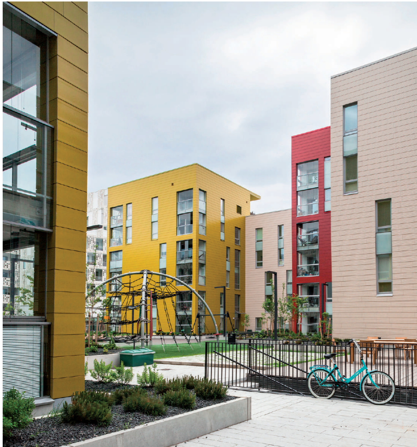
tempio® [projects] Saukonkanava, Helsinki, Finland.
